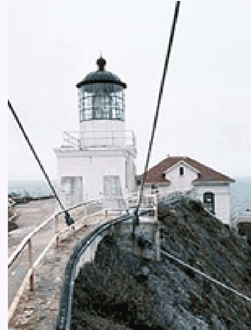
U.S. Coast Guard lighthouse with beacon antenna.
